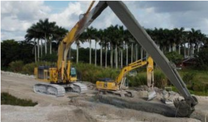
Figure 18: Self-Hardening CB (Cement-Bentonite) Slurry Wall Method (Geo-Solutions, 2025)
